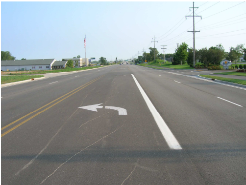
Previously Completed Section
