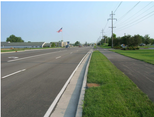
Previously Completed Section
