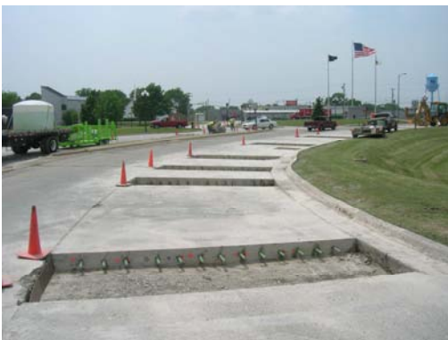
Concrete Pavement Patching
